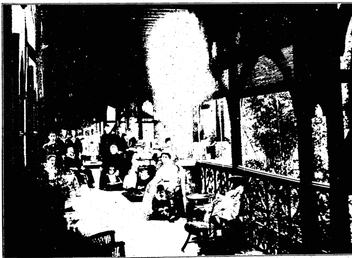
WEST VERANDAH, CONVALESCENT HOME, KHANDALLA.
